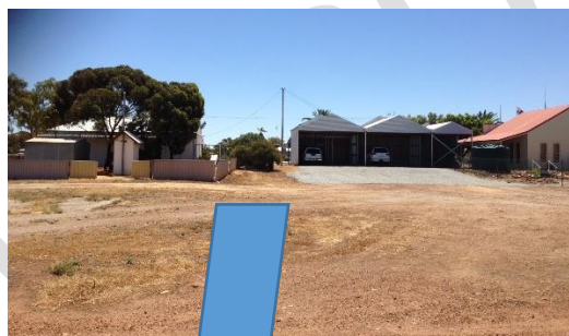
Admin Carport/CWA building rear
